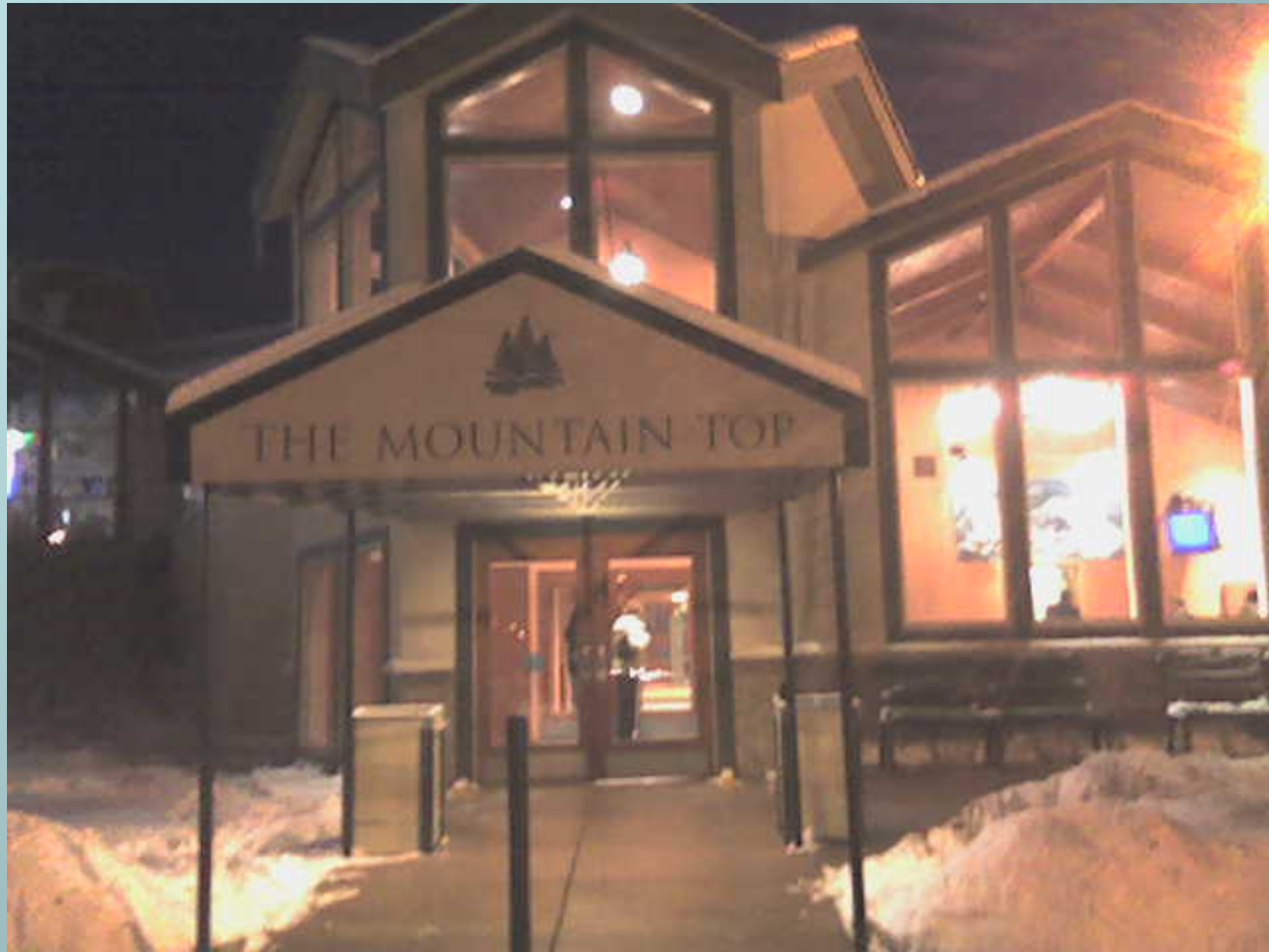
Entrance to the Mountain Top from the Parking Lot
